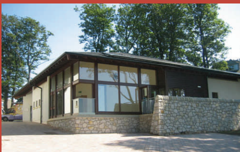
- Paxton Centre, Lundin Links viewed from the South -
